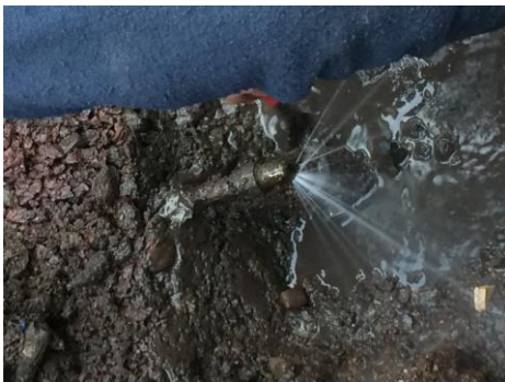
First leak excavation
