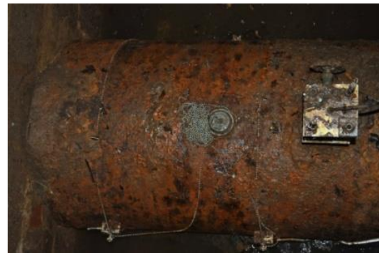
Sensors installed on 600mm ductile iron pipe
