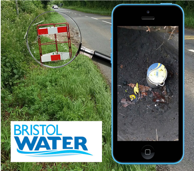
Enigma installation next to the A4135 highway
