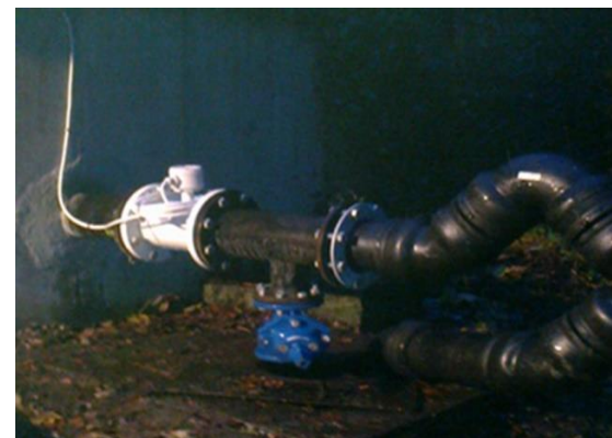
Flowmeter installation
