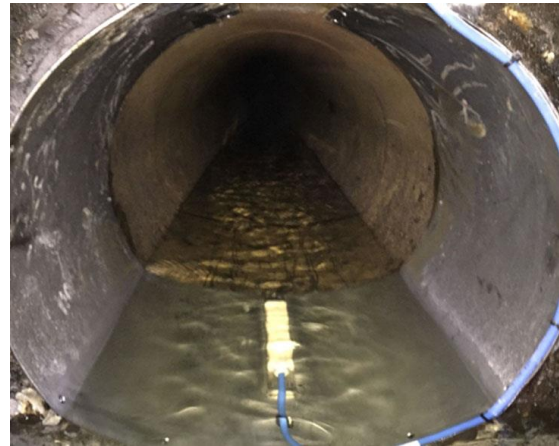
Doppler sensor installation
