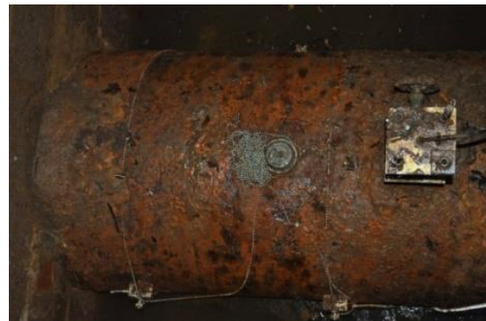
Sensors installed on 600mm ductile iron pipe
