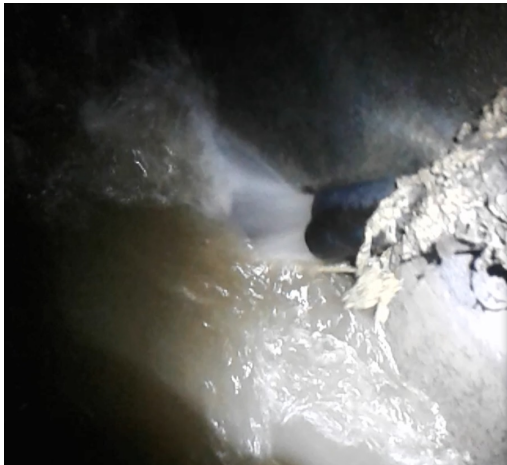
Faulty valve releasing water to waste water system
