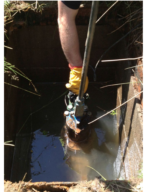
Enigma-hyQ logger installed on 500mm PVC main via fire hydrant
