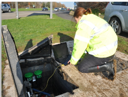
Bristol Water installation
