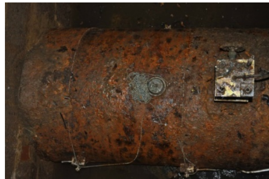
Sensors installed on 600mm ductile iron pipe
