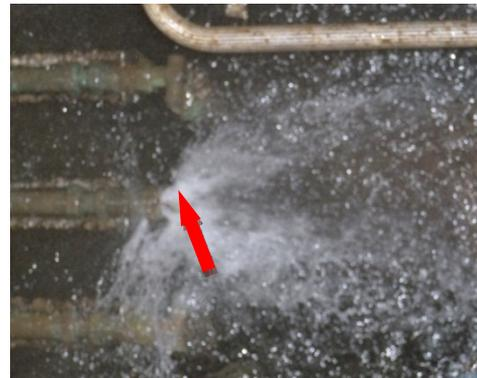
The leak identified at valve shut 9.
