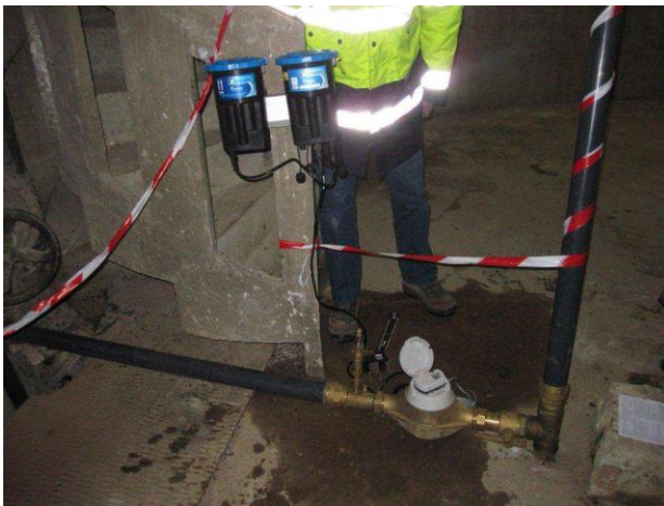
By-pass with meter and Xstream installed
