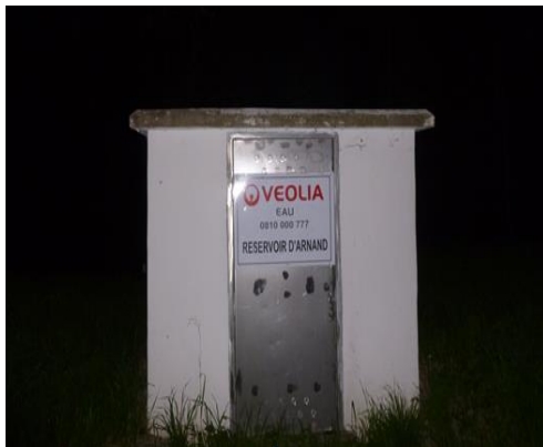
The tank supplying the sectorized network.
