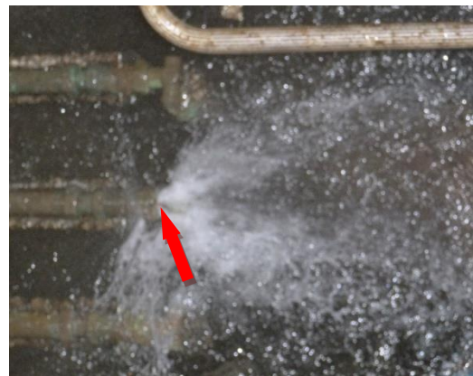
The leak identified at valve shut 9.
